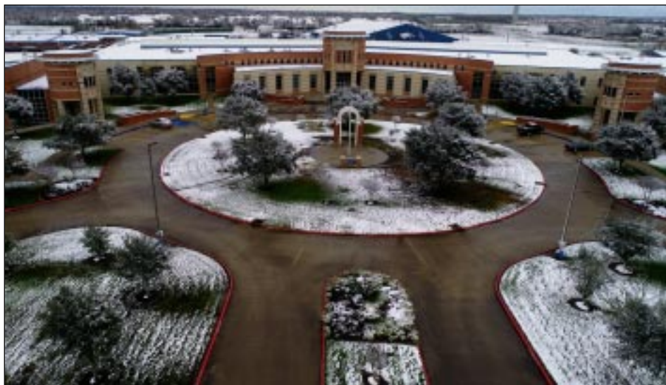
Barbers Hill ISD recently reconstructed at the current high school the original arch from the 1930 Barbers Hill High School. District officials estimate that 877 Barbers Hill graduates passed under these arches when the building served as a high school. This photo was taken December 8, during the district's late arrival Snow Day.
