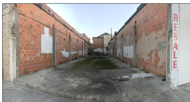
The alley prior to improvement.
