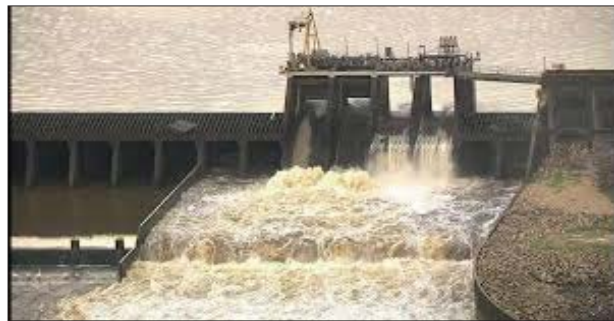
Lake Houston spillway opened.
