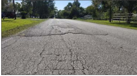
Road improvements in Lynchburg area.
