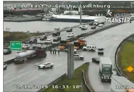
TRAFFIC WESTBOUND at 4:33pm was blocked by TxDOT trucks and the police, as engineers assessed the damage. Later one lane was opened, and on Tuesday two lanes, but the on-ramp from Crosby-Lynchburg was closed, causing massive backups from Highlands to Crosby and Baytown. (Transtar Photo)
