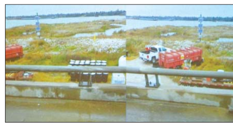
SAMPLES of ground water, and cores are being stored in these drums, and then taken off-site for lab tests to determine the toxicity of the material under the cap, and how high the water table is below.
