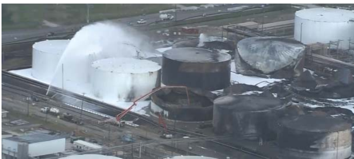
CLEAN-UP continues at the ITC site in Deer Park. In this photo, taken over a week after the fire, foam is being sprayed to seal tanks, and a pump truck at center is removing chemicals that still pose a hazard. (Photo courtesy KPRC)
