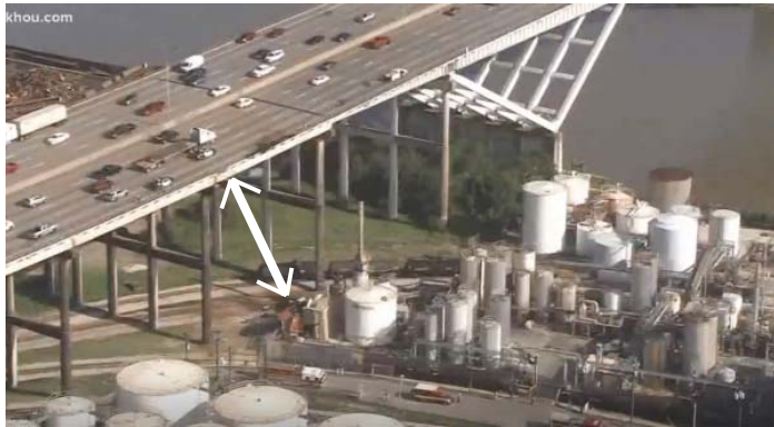
ANOTHER TRUCK ACCIDENT is seen in this view, of an 18-wheeler that went over the side of the I-610 East Loop bridge over the Houston Ship Channel. The top of the arrow marks where the truck broke through the rail after swerving after hitting a car that cut in front of him. The bottom of the arrow shows where the truck landed on top of a chemical building at Huntsman Chemical, 150 below the bridge. The driver of the rig died pinned in his cab, as rescue workers tried to extract him.
