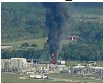
The flames that evacuated over 200 neighbors after they had flooded.
