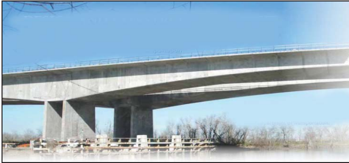
TxDOT engineers have said that the bridge design will be segmented, similar to this design of IH-10 over the Trinity River. The center span is 450 feet, so that support columns do not need to be in the river.
