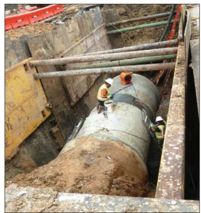
NEW SECTIONS OF 96" STEEL PIPE ARE BEING INSERTED INTO THE BREACH.
