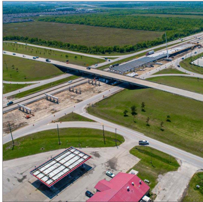
Aerial view of FM 3180 and I-10 intersection where construction is ongoing.
