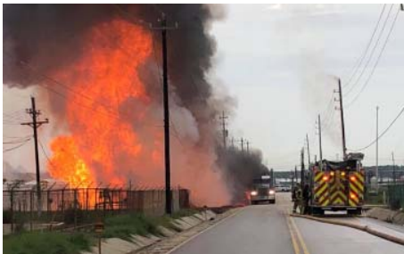
First on the scene, Mont Belvieu Fire Dept. arrived shortly after 4:50 p.m. to stop the spread of flames from a wellhead said to have begun when a contractor hit a pipeline.
