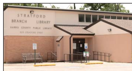
STRATFORD LIBRARY in Highlands
