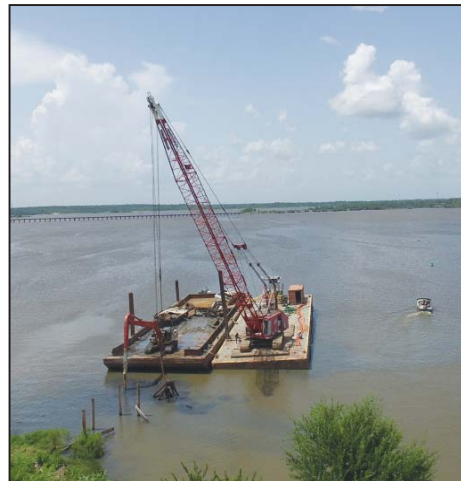
Two GLO contractor's work barges, with cranes and excavators, lifting portions of sunken barges.
