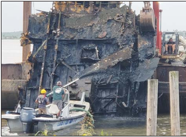
Workers clean mud off barge that has been raised from underwater.
