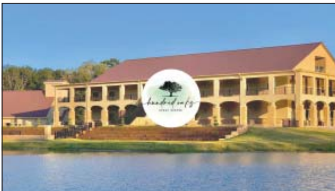
The Hundred Oaks Event Center main building, with the Chapel to the left and the outdoor Belvedere ceremonial site and lake in front. The re-opening will take place on November 30 with a ribbon cutting at noon.
