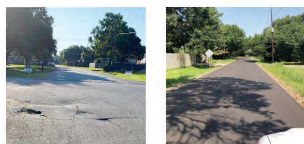
Precinct 3 released these photos, showing what the reconstructed road will look like before and after the asphalt repairs.
