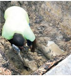
Utility workers repair leaking pipes at Newport, that are contributing to the problem of limited capacity at the water treatment plant.
