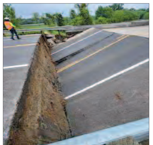
TSCOT examines Hwy FM787 for repairs.
