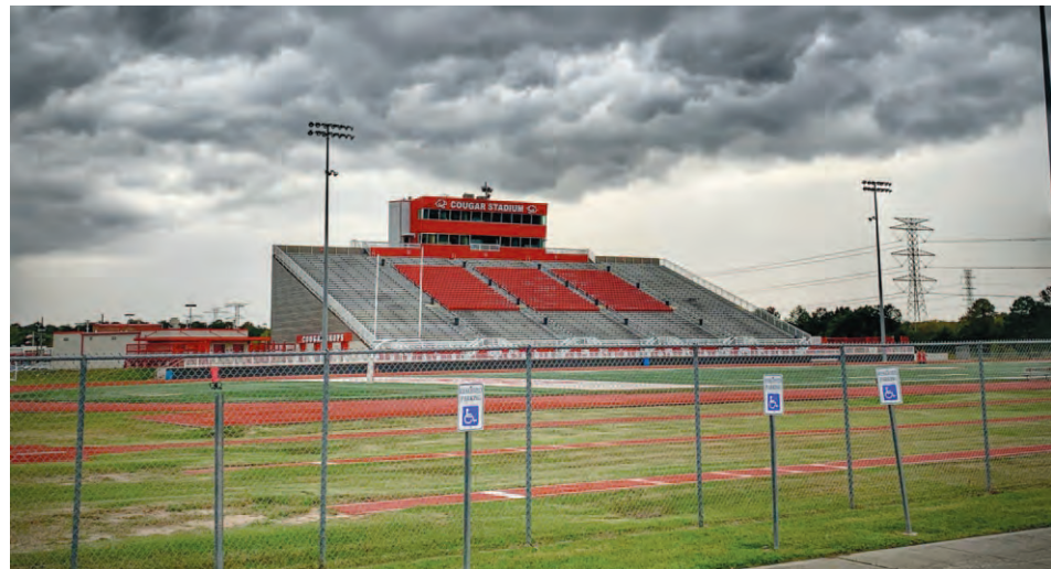
Cougar Stadium will undergo turf replacement this summer. The stadium was closed to the public starting June 3rd.
