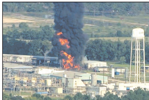
The Arkema chemical plant in Crosby had multiple fires and explosions, due to flooding and power failure of refrigerated chemicals.
