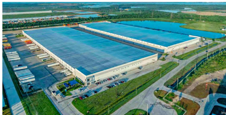
Aerial View of Ikea's warehouse in the Cedar Port Industrial Park
