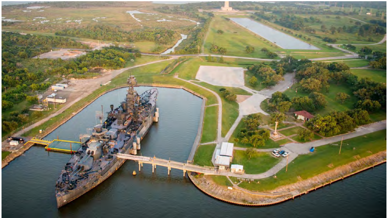
The berth dredged to house Battleship Texas, seen here in 2013, will be restored to its original landscape. Photo credit Smiley N. Pool/Houston Chronicle via Getty Images
