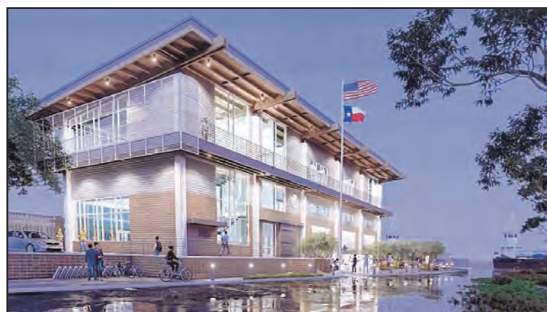
The new Lynchburg Ferry Operations Building will be 3 stories tall, 14,000 square feet, equipped with flood walls and gates, and cost $21 million dollars. (PBK architects).
