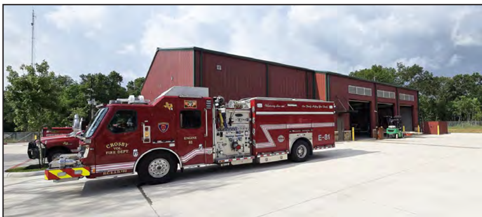
The new maintenance facility for the Crosby Volunteer Fire Department sits behind Station 82 and will help service the 45 vehicles in the fleet.
