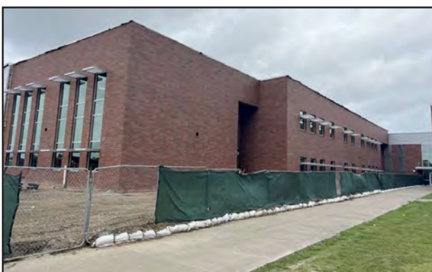
The Crosby High School expansion includes new state-of-the-art welding and carpentry labs. The expansion will open this fall as the Gray House, joining the Red House and White House at Crosby High School.
