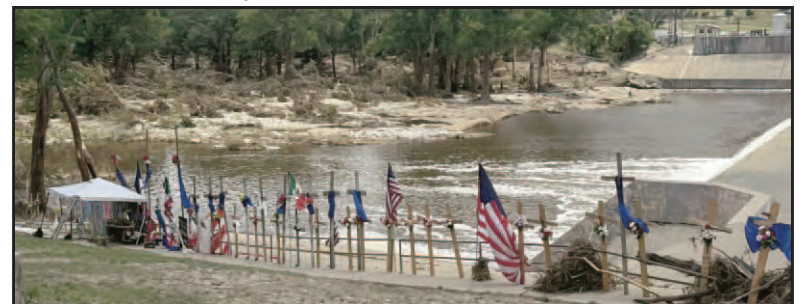
A View of the Flood Damage and washed-out foliage along the Guadalupe River
