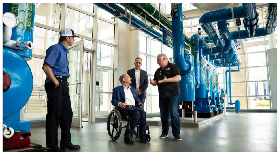
Abbott received a tour of the facility from IUOE management prior to his press conference touting the new jobs council and Texas achieving No. 1 status for producing the most jobs in the nation.
