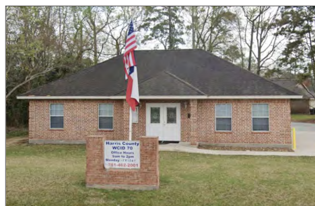
Harris County WCID70 Office Building
