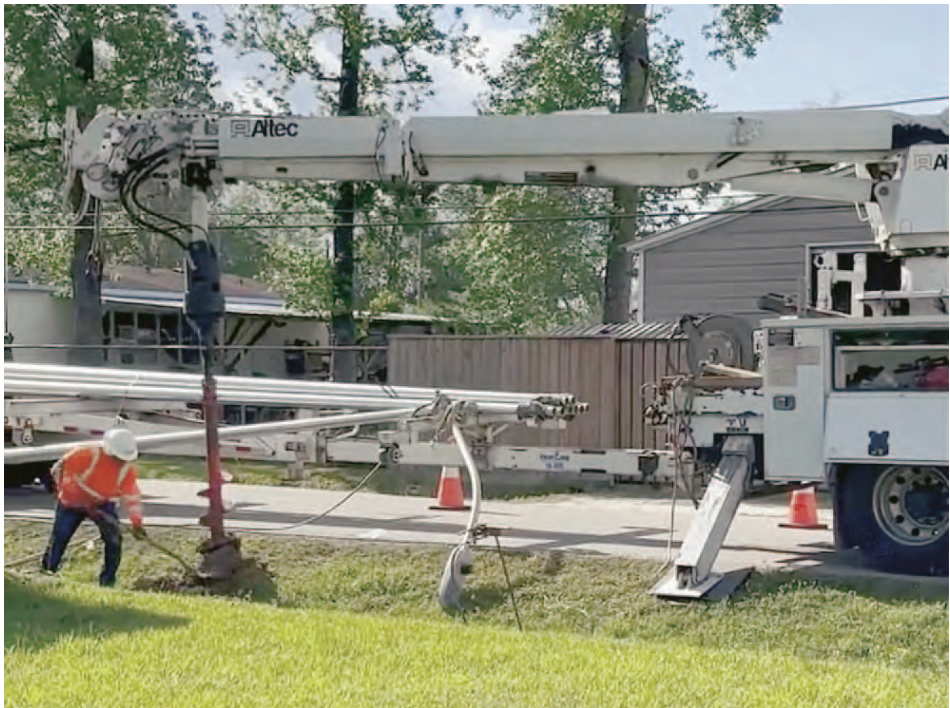
A utility crew installs one of the nearly 600 new street lights in Barrett Station.
