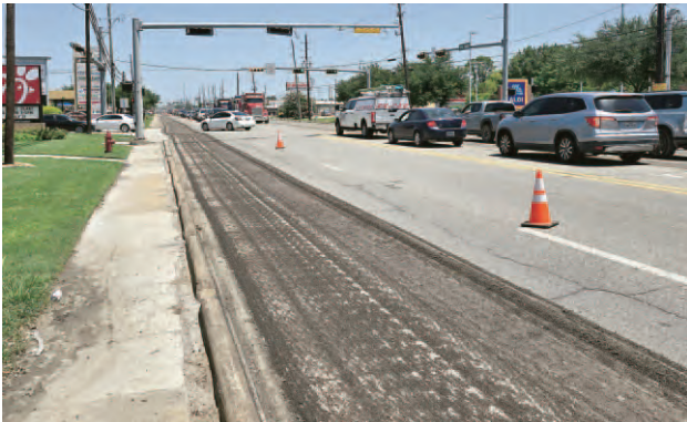
By Monday, much of the paved lanes on both sides of FM 2100 had been milled in preparation for a new overlay of asphalt later this week. Contractors at Forde Construction hope to finish the work before the start of school.
