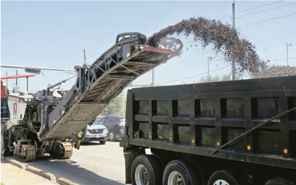
A large dump truck precedes cold milling machine or cold planer to mill up the pavement using a large rotating drum equipped with carbide-tipped teeth to grind up asphalt or concrete. The planer features a conveyor belt to dump the debris directly into haul trucks for recycling.
